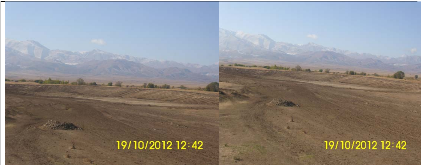
Mechanical rehabilitation of loam quarry «Land lot-3»
