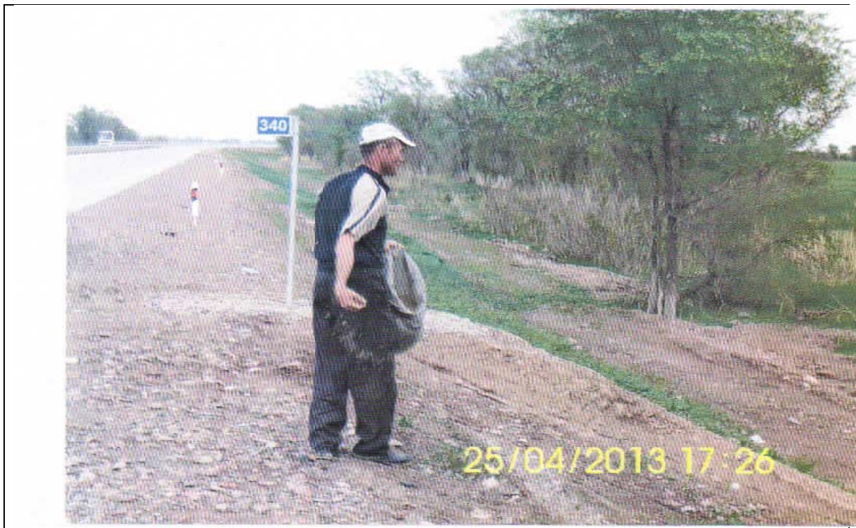
Biological Rehabilitation on shoulders-of road section km 356.8-389.4
