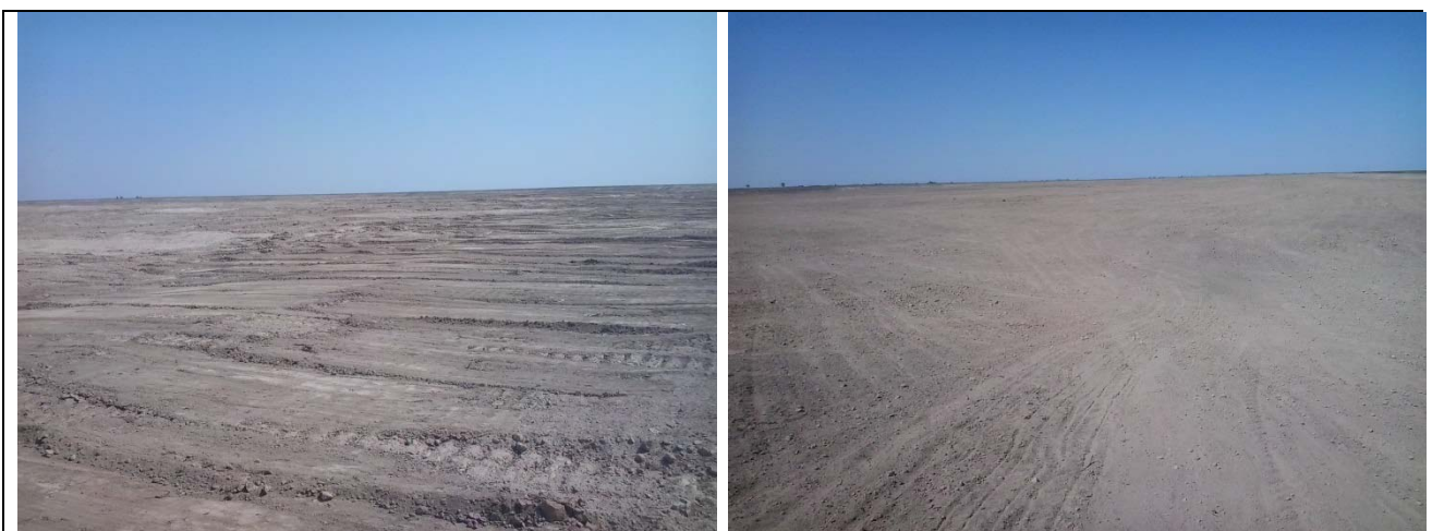
Rehabilitation Works on Quarries – RysKulovskyi
