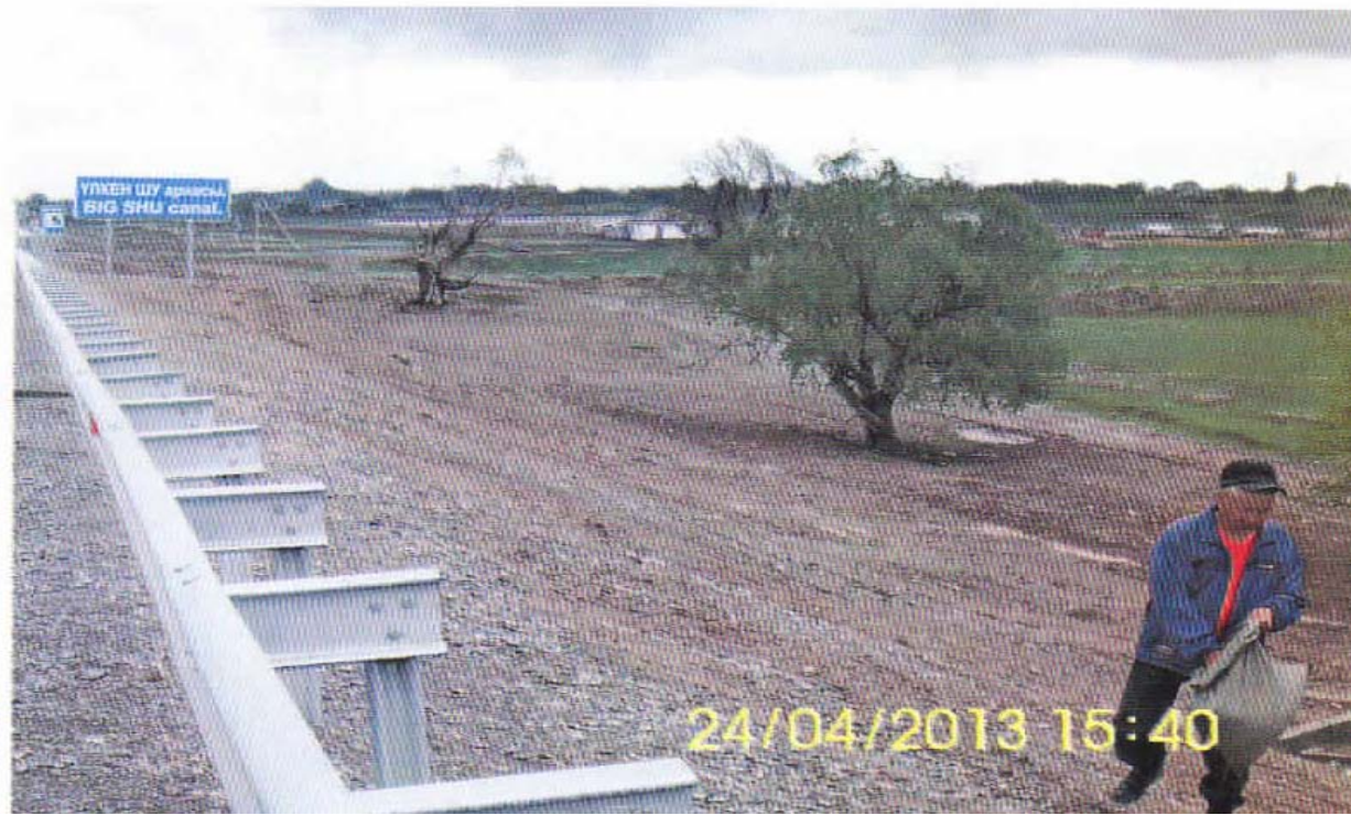
Biological Rehabilitation on shoulders-of road section km 356.8-389.4 (Big Chu Channel)
