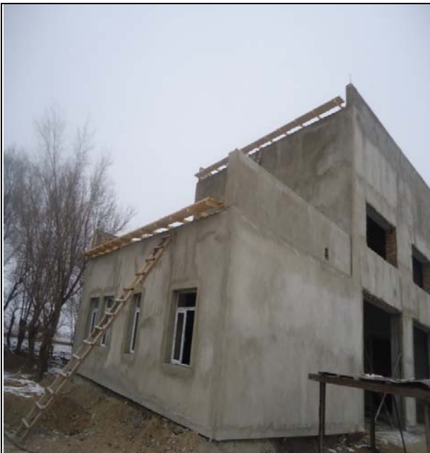
Maintenance depot-v.Otar, Repair Workshop- Roofing
