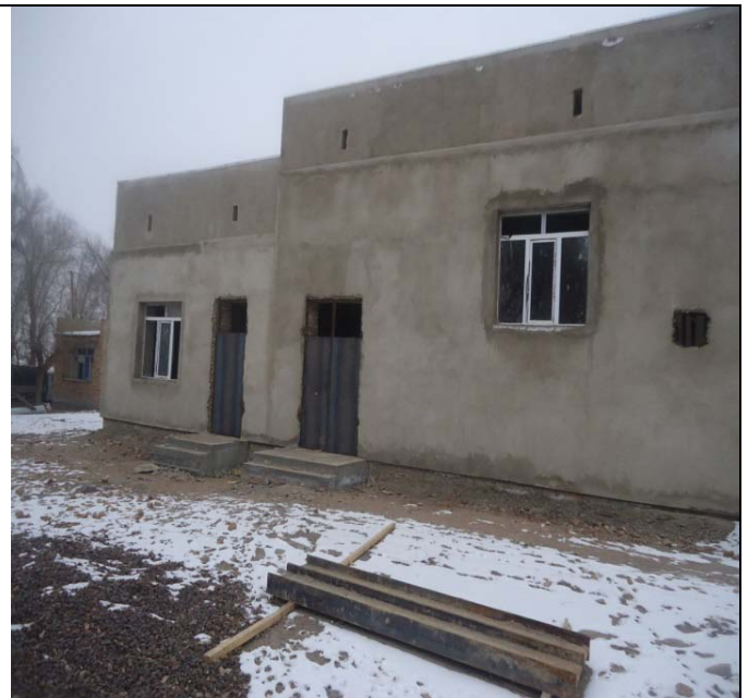
Maintenance depot-v.Otar, Boiler House- Roofing
