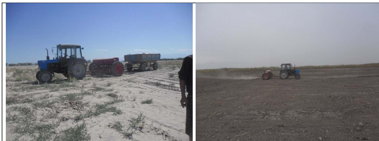
Rehabilitation works on Quarries – Aspara 1 (Left) and Aspara 2 (Right)
