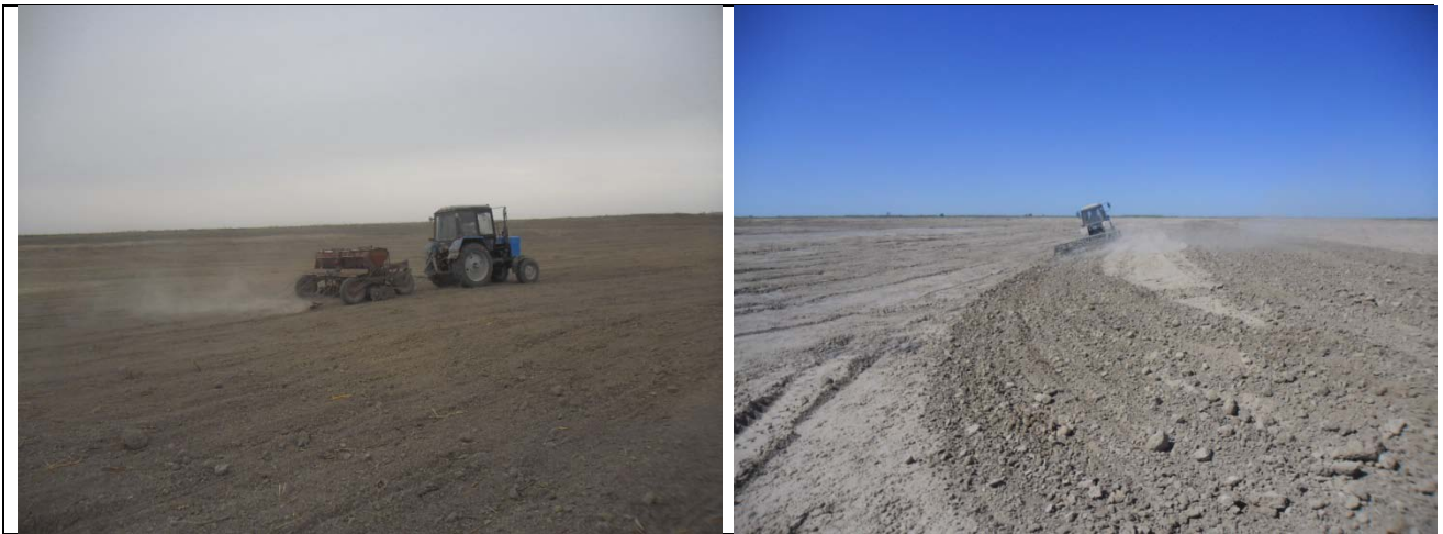
Rehabilitation Works on Quarries- – Kuruzek (Left) and Kuralas (Right)
